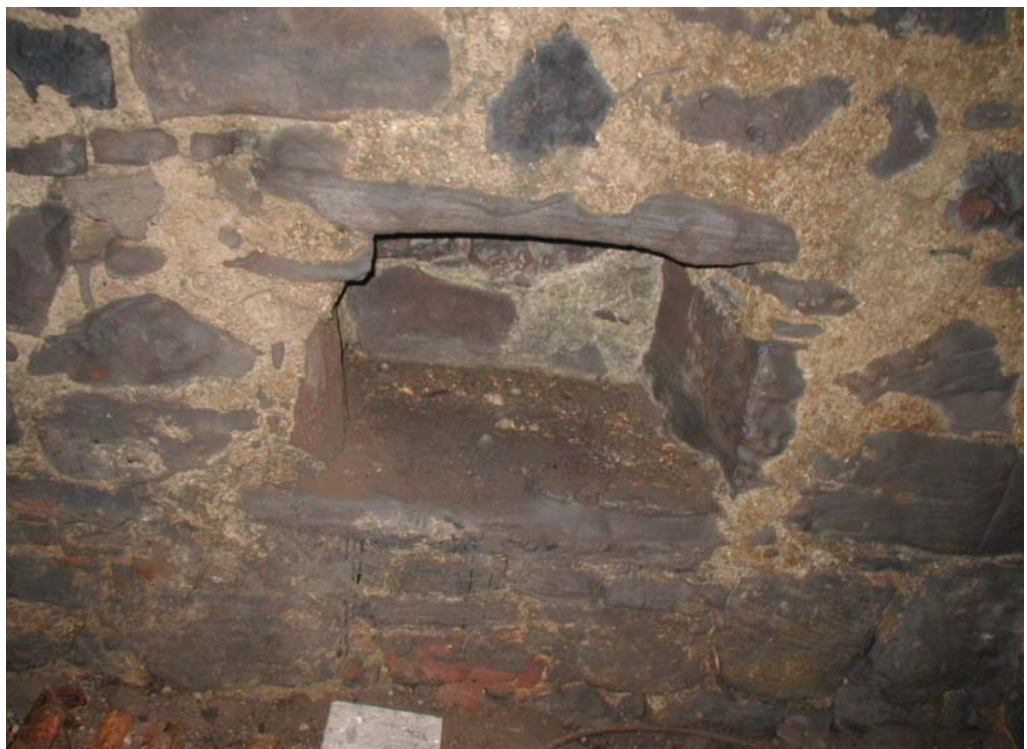
Figure 43: Cupboard Feature A-S: L
