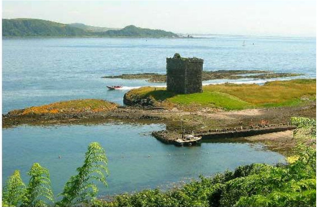
Figure 49: Portencross from the North (SCRAN)
