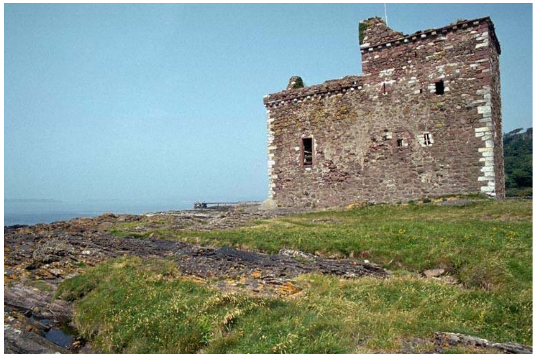
Figure 3: South elevation (SCRAN)
