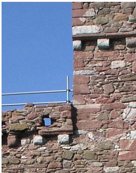
Figure 36: Corbelled moulding A-S:L
