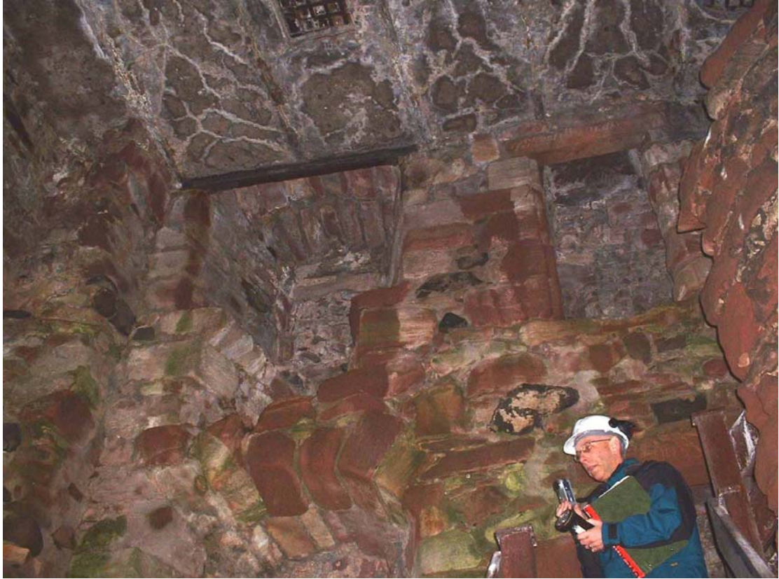
Plate 55: Window W3-2, Garderobe (D3-3) and concrete roof.
