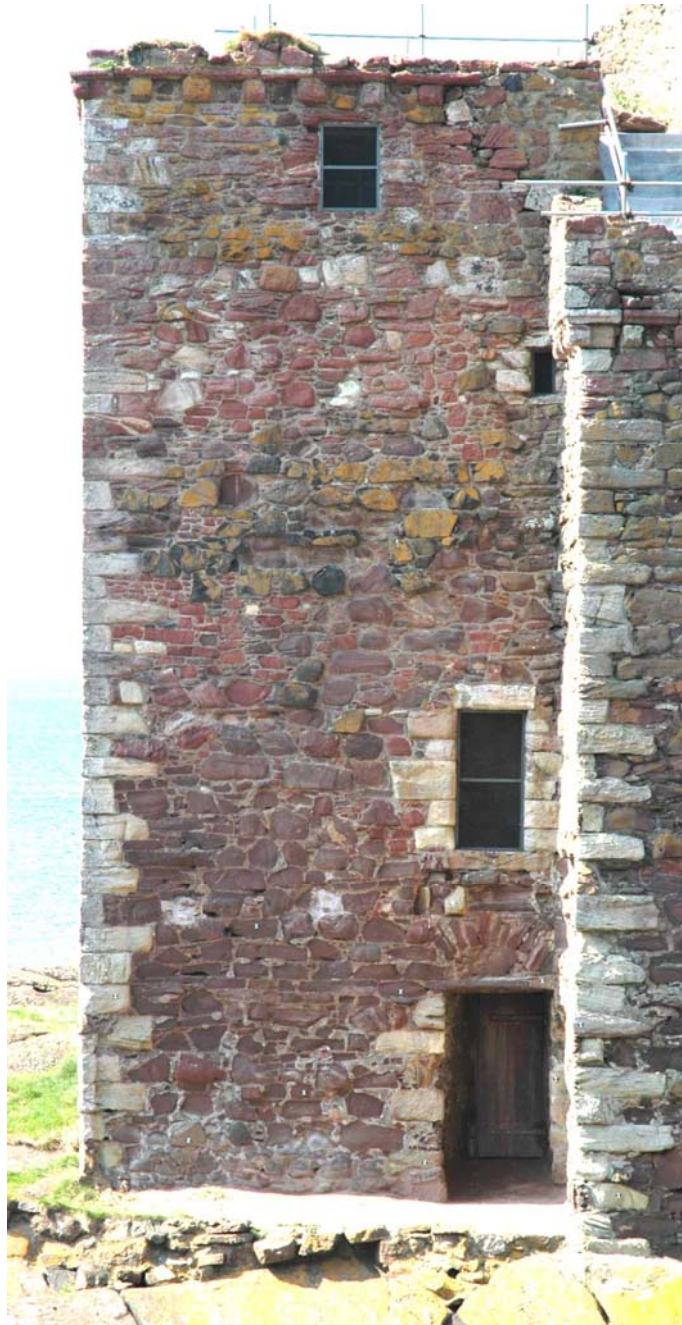
Plate 30: Elevation 16, north-east facing.
