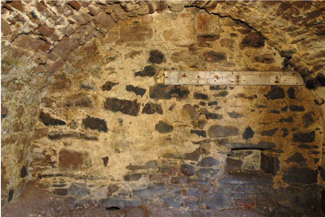
Plate 37: Cellar wall 110, see drain left, off centre.
