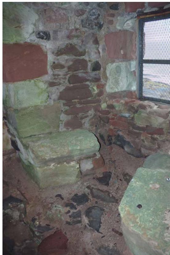
Plate 52: Window W2-2 with benches.
