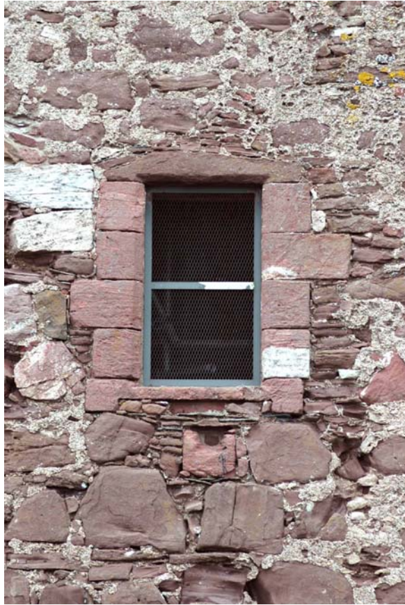
Plate 20: Window into Spiral stair W1-4.
