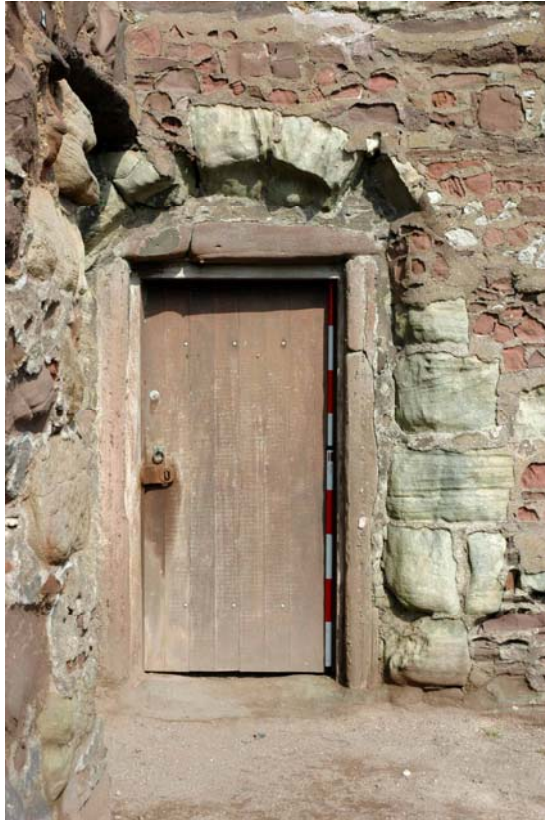
Plate 8: Ground floor doorway DG-1.
