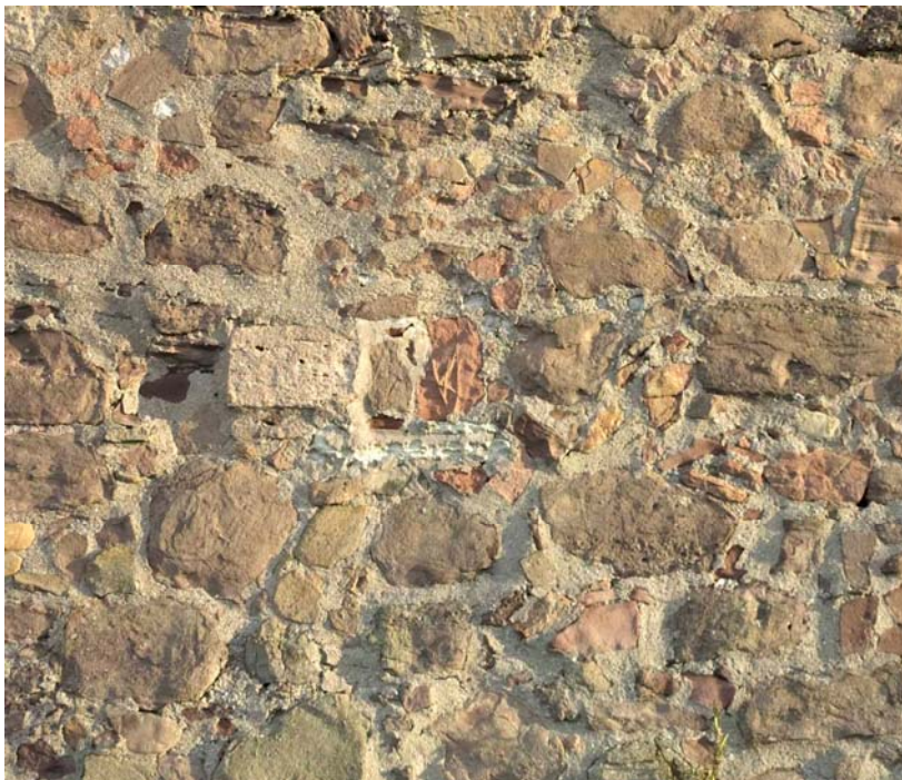
Plate 19 Blocked window into pit prison, 071.
