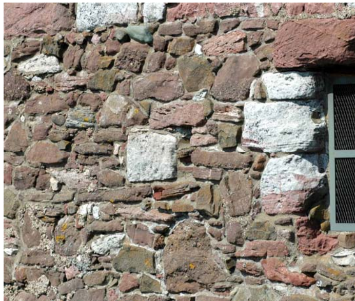
Plate 23: Possible blocked opening 079.
