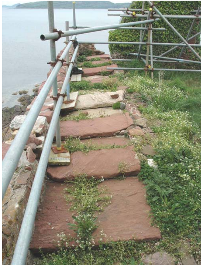
Plate 57: Lower Roof parapet walk with saddle and trough drains.
