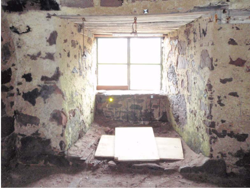
Plate 39: Inserted window WG-3 internal.
