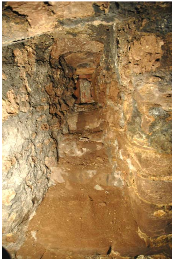
Plate 42: Blocked window WG-2.
