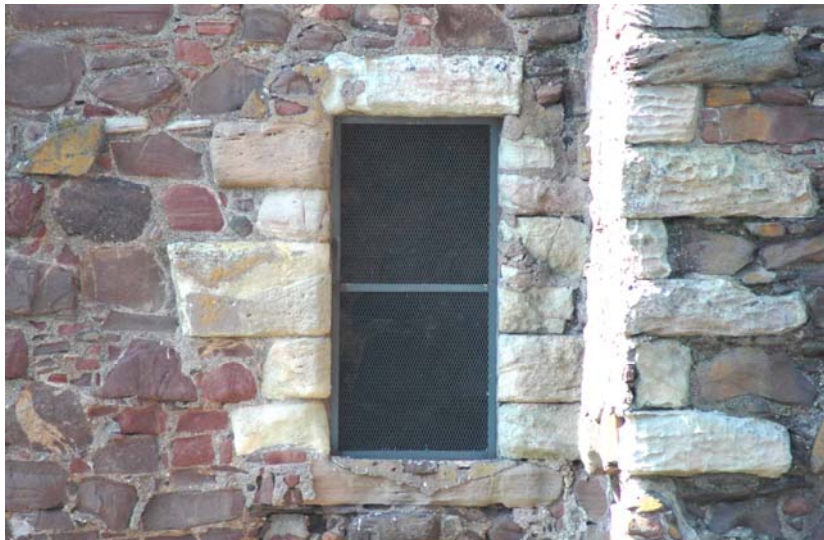
Plate 32: Window W1-1, possibly an earlier doorway.
