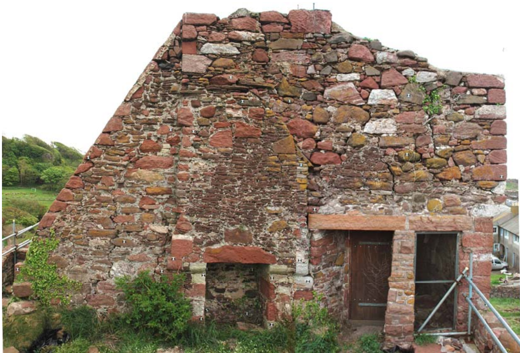
Plate 56: Gable of Lower roof (see Figure 15).
