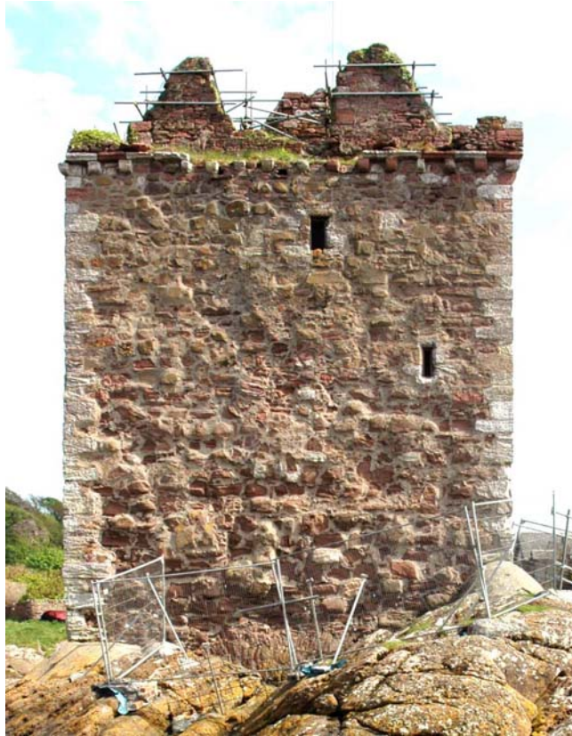
Plate 26: Elevation 4, north-west facing.
