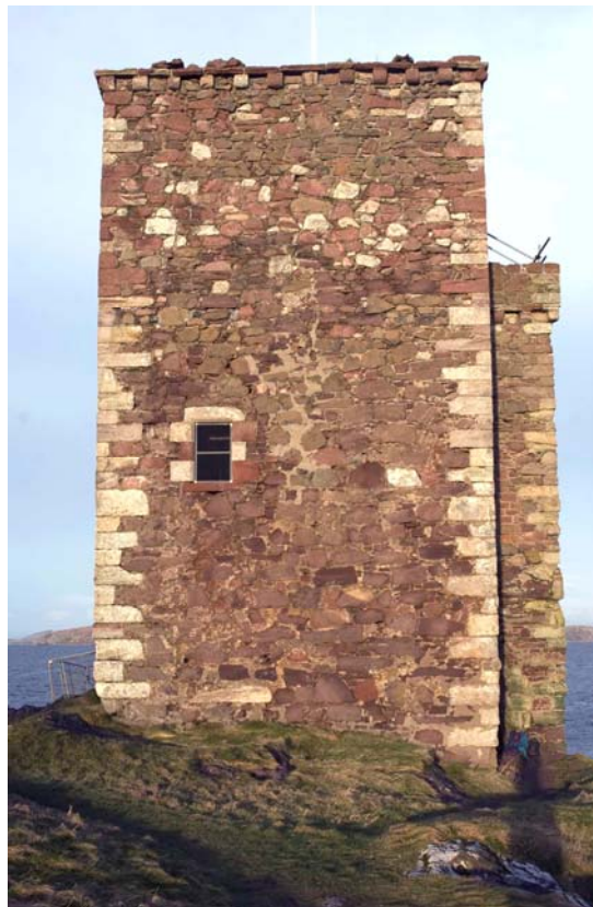
Plate 13: Elevation 2, south-east facing.
