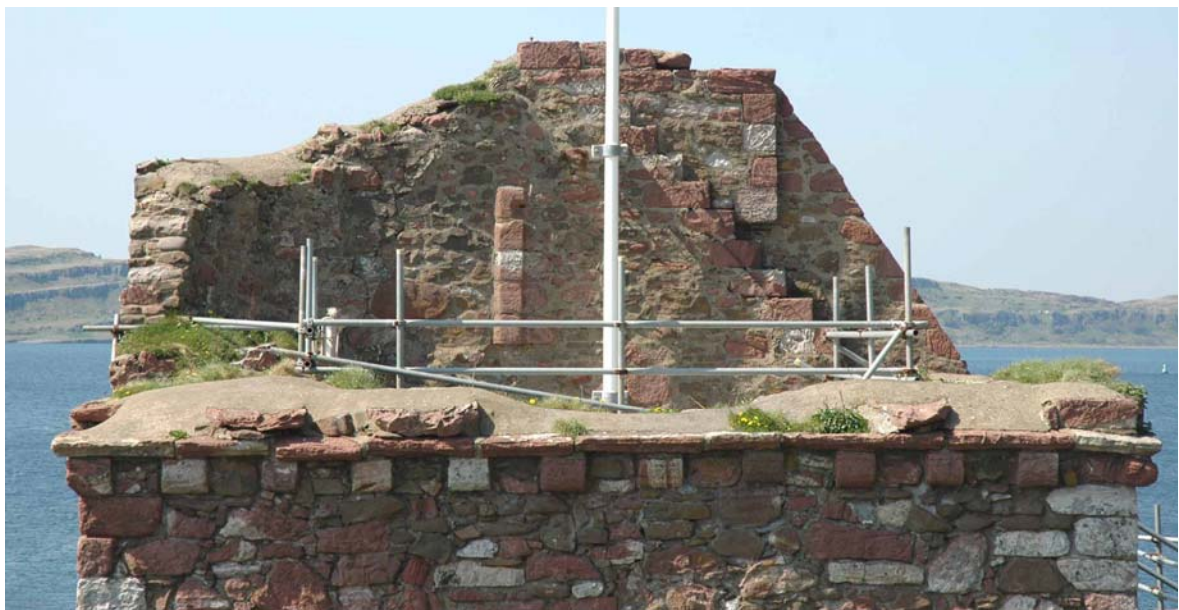
Plate 58: Gable of Upper Roof.
