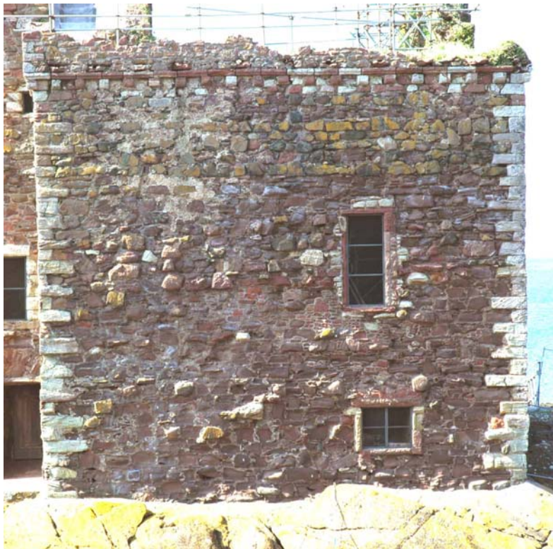
Plate 9: Elevation 1, north-east facing.
